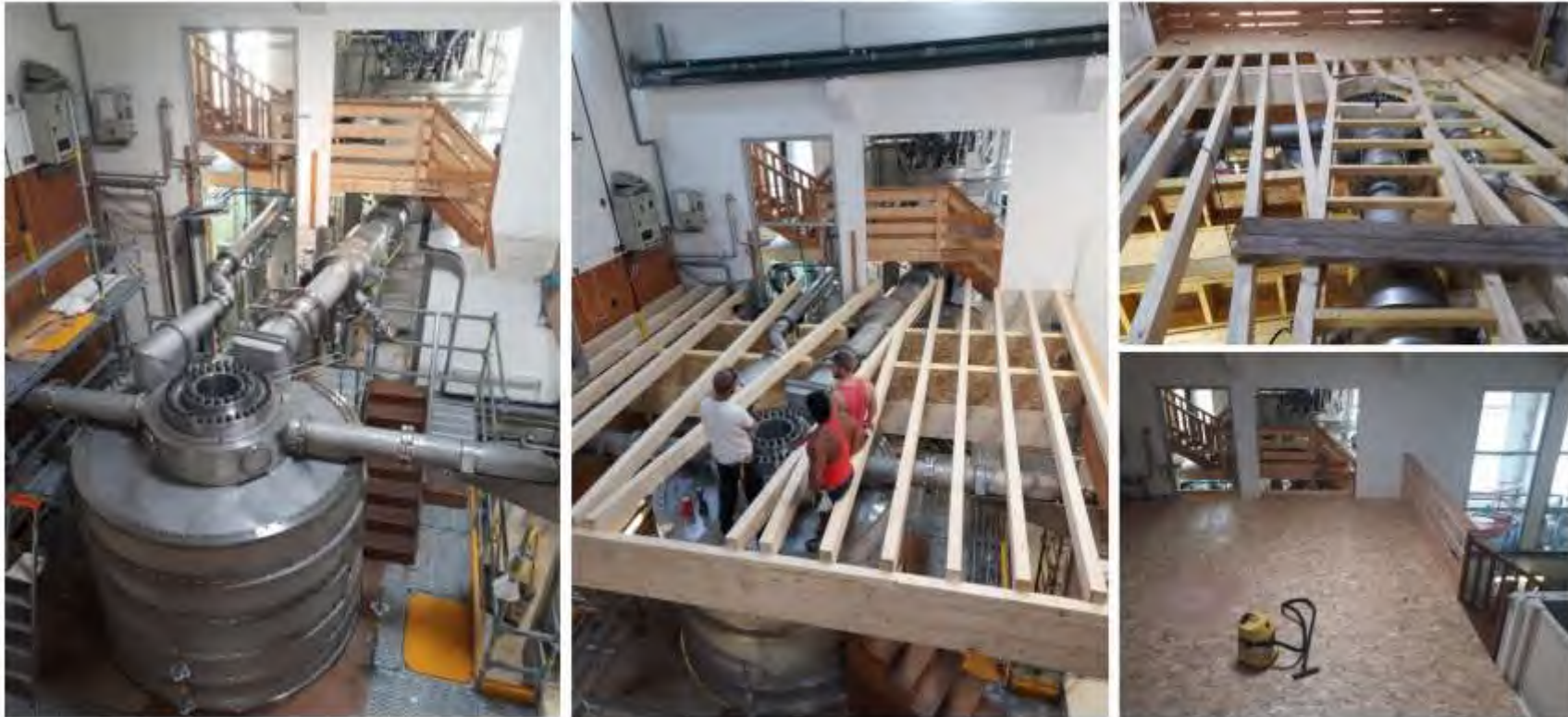
Mounting of the mezzanine for users (May 2022)
