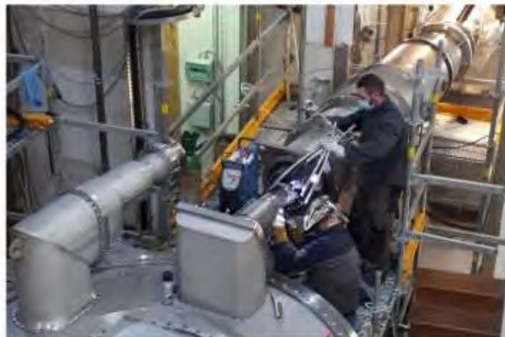
Welding of the cold mass of the cryogenic line to the magnet one
